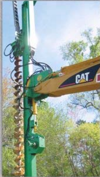
Set up for pile predrill
