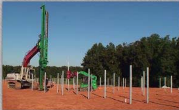
Solar field foundations
