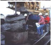
with the excavated spoils and then redrilled the same day with KB's CDP System and an auger.
