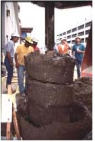
possible to slurry-drill with augers, even in sand and gravel, often eliminating the need to use a bucket. This feature can reduce drilling time, increase productivity and reduce slurry wastage.
