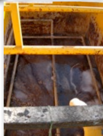
Steel Tube Aeration Lines Running the Length of a Slurry Storage Tank
