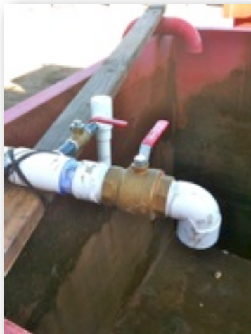
Ball Valve Connected to Casing
