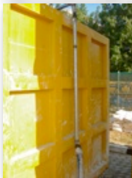
Steel Tube Aeration Tube Being Run Over the Side of a Storage Tank
