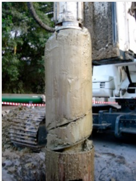
Example of Actual Solid Clay Loaded Auger which Collapsed Pile due to Piston Effect and Suction
