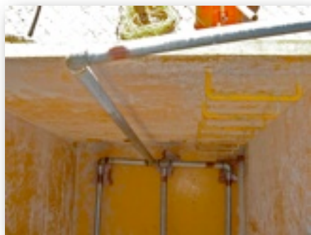
Steel Tube Being Run Over the Side of a Storage Tank and Divided into Aeration Lines
