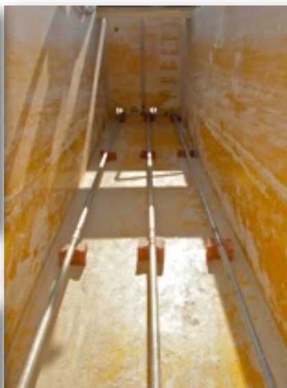
Steel Tube Aeration Lines Running the Length of a Slurry Storage Tank
